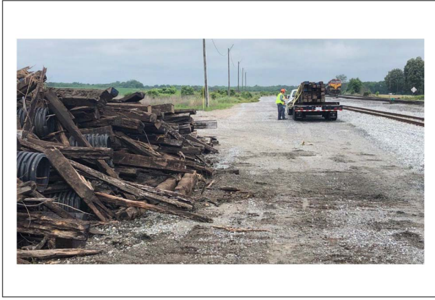
Figure 2.—Collection of legacy ties at a commercial railroad stockpile.
