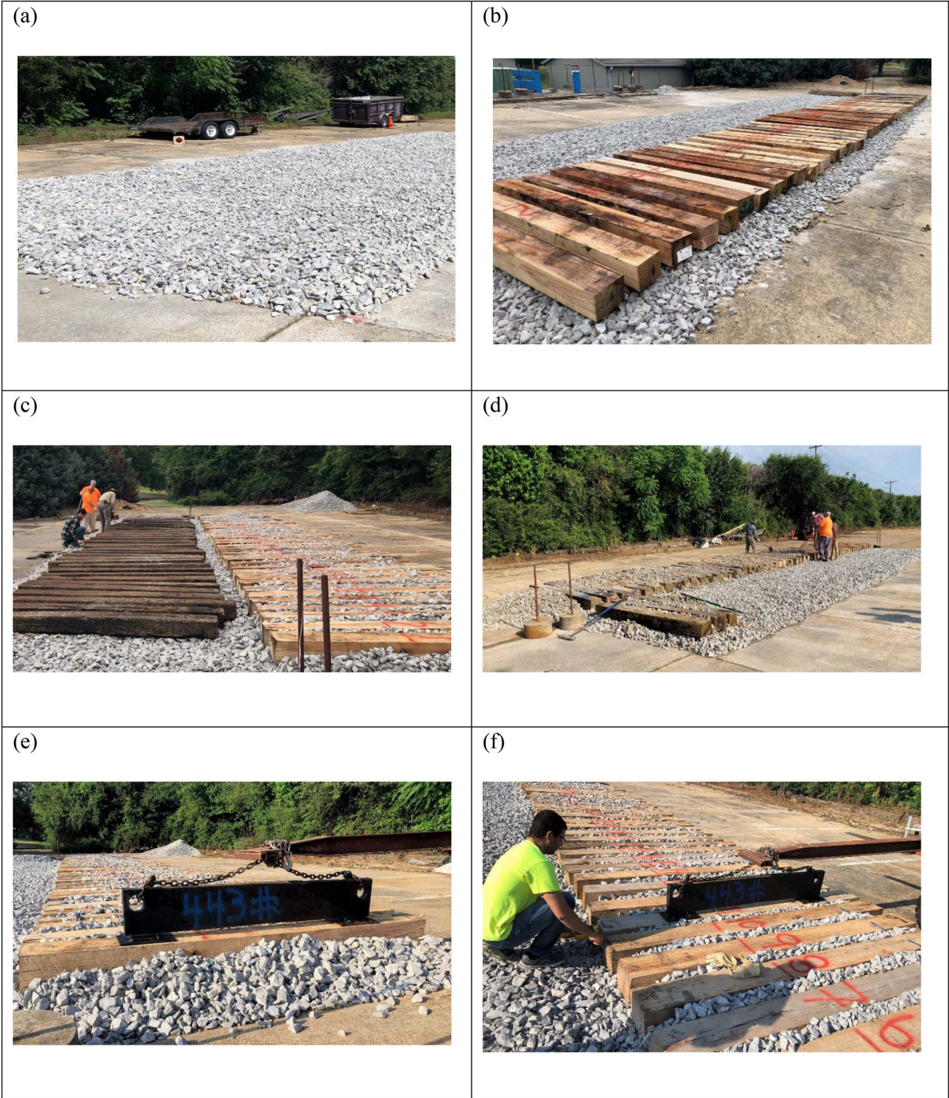
Figure 1.—(a) Ballast rock bed, (b) freshly cut green ties installed on the ballast, (c) installation of legacy ties on the ballast, (d) installation of ballast between each of the ties, (e) 200-kg (434-lb) weight constructed and used to simulate the load of the rails on each tie, and (f) measurement of acoustic velocity of a given tie (identification number 11) while in the fixed boundary condition.
