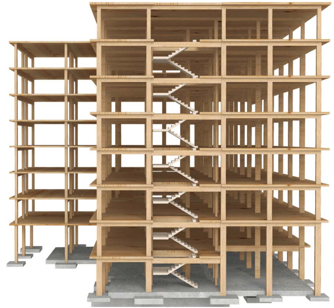
Rendering of the first Type-IVC IBC Building Code building permitted in the City of Seattle. Photo courtesy of atelierjones.
