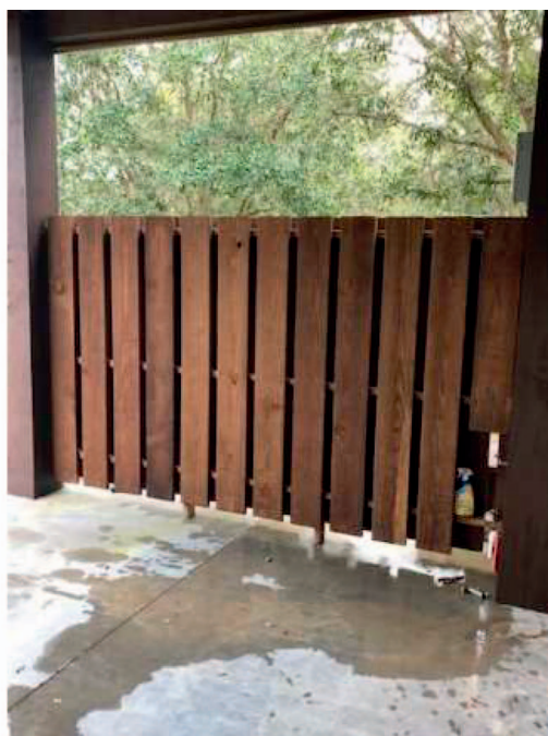
Figure 5.—No checking on chromated copper arsenate/oil-treated fence boards on the exposed (left) or protected (right) side after more than 8 years of exposure.
