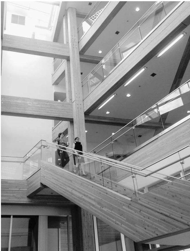
Figure 3.—Example of architectural elements (engineered timbers); University of British Columbia CIRS Building. Photo by C. Gaston.
