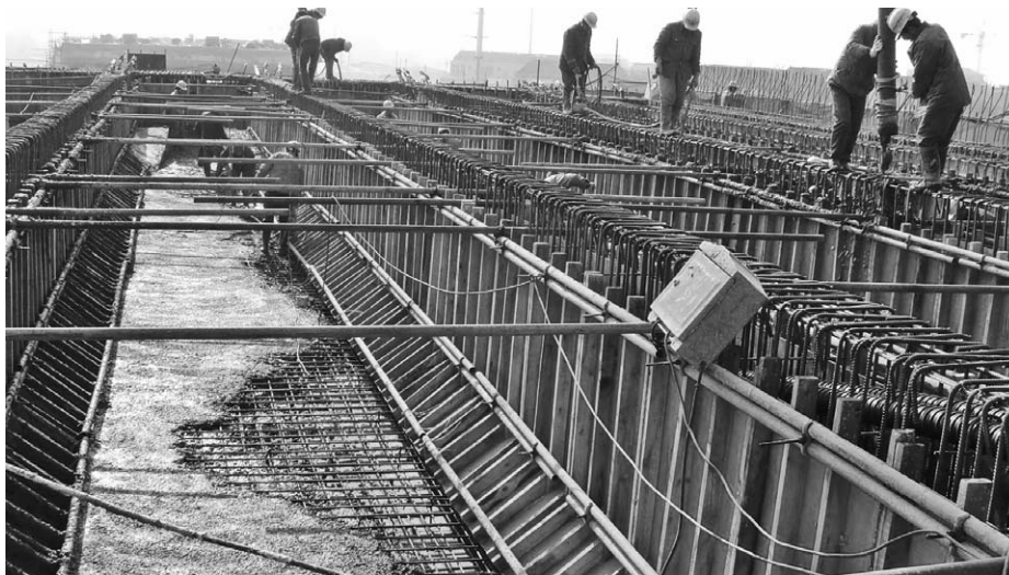
Figure 4.—Concrete form construction in China (Fang 2013).
