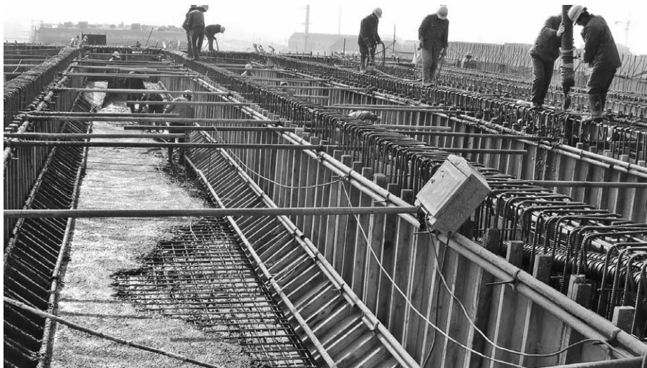
Figure 4.—Concrete form construction in China (Fang 2013).
