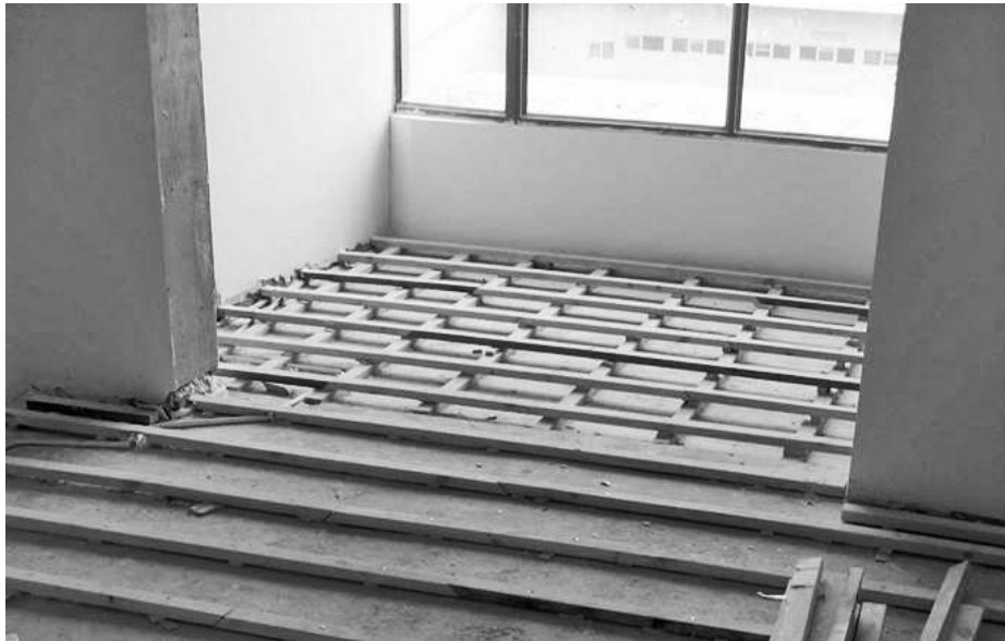
Figure 5.—Furring strip flooring lattice framework (Owen 2012).
