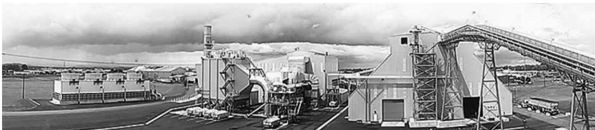
Figure 2.—Seneca Sustainable Energy Cogeneration plant, May 27, 2011. Photo courtesy of Seneca Sawmill Company.
