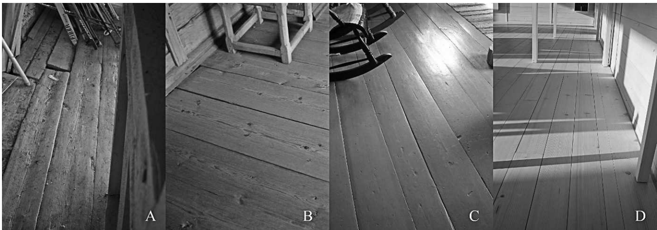
Figure 7.—Finnish wood floors from the end of 19th century (A) to the beginning of the 21st century (D). The two oldest floors on the left (A and B) do not have any surface treatment. The floor in C is painted, and the floor in D is finished with lye and oil.
