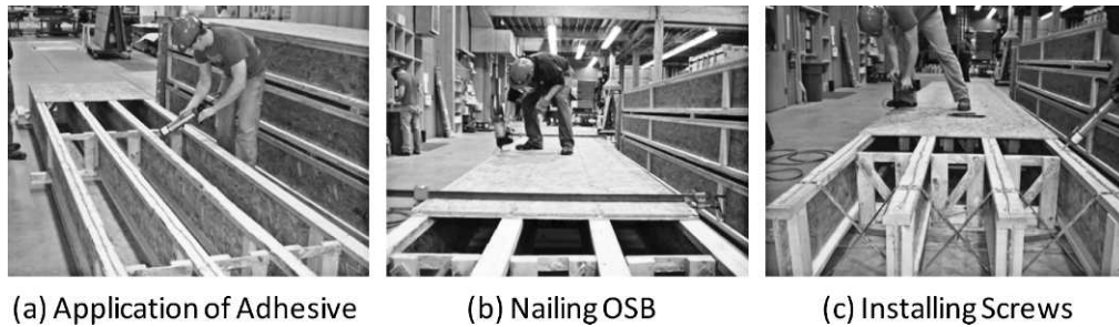
Figure 3.—Panel fabrication. OSB = oriented strand board.
