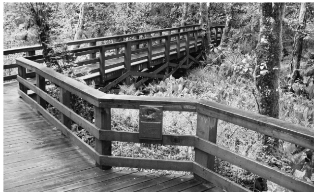
Figure 1.—Test section of boardwalk 11 years after construction. Soil samples were removed from the area in the foreground of this picture, while sediment samples were removed adjacent to the elevated walkway in the background.
