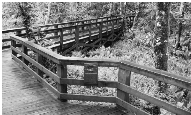
Figure 1.—Test section of boardwalk 11 years after construction. Soil samples were removed from the area in the foreground of this picture, while sediment samples were removed adjacent to the elevated walkway in the background.
