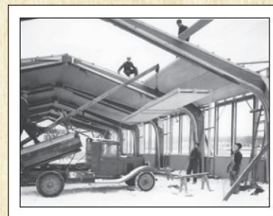
Glued-laminated (glulam) beams and arches use multiple layers of lower-grade wood to create large durable beams.
